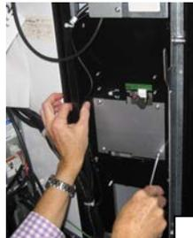
Remove the Blocker Plate (save the 4 screws)
